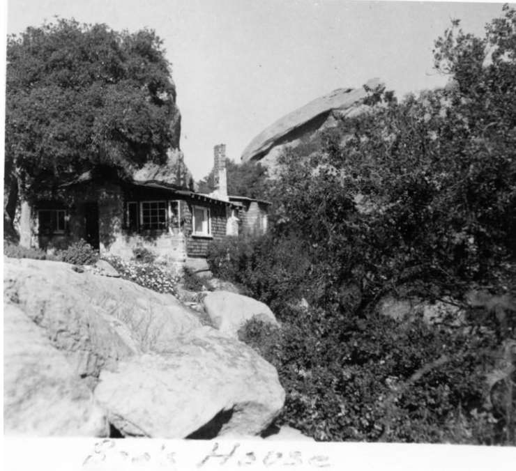
Bee's House Figure 21 View of the SW corner of house
