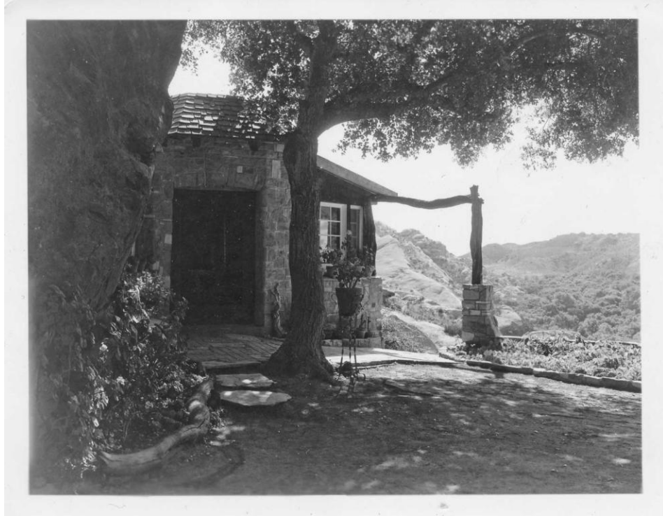
Figure 9 Front (west) side of house (2)
