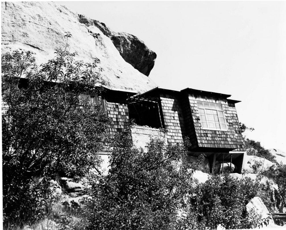
Figure 6 Canyon (south) side of house
