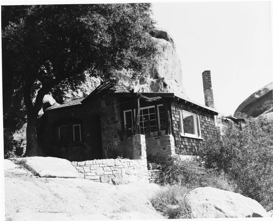
Figure 8 View of SW corner of house: photo by Universal Pictures
