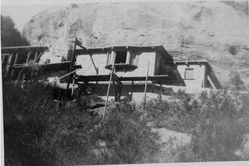
Figure 5 Canyon (south) side of house under construction
